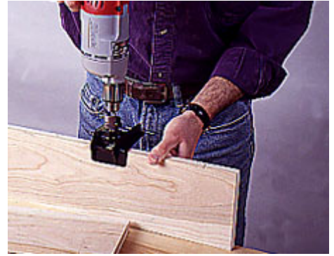
3 -Using small dowels helps with edge joint alignment. Bore the dowel holes with a doweling jig and an electric drill.
